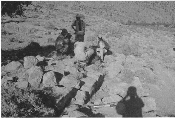
Plate 11.31 Tang-e Bolâghî: a stone lining constructed as the sidewall of the road.
